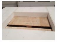
As the panels are easily cut, both edges of the corners can be cut at a 45-degree angle.
